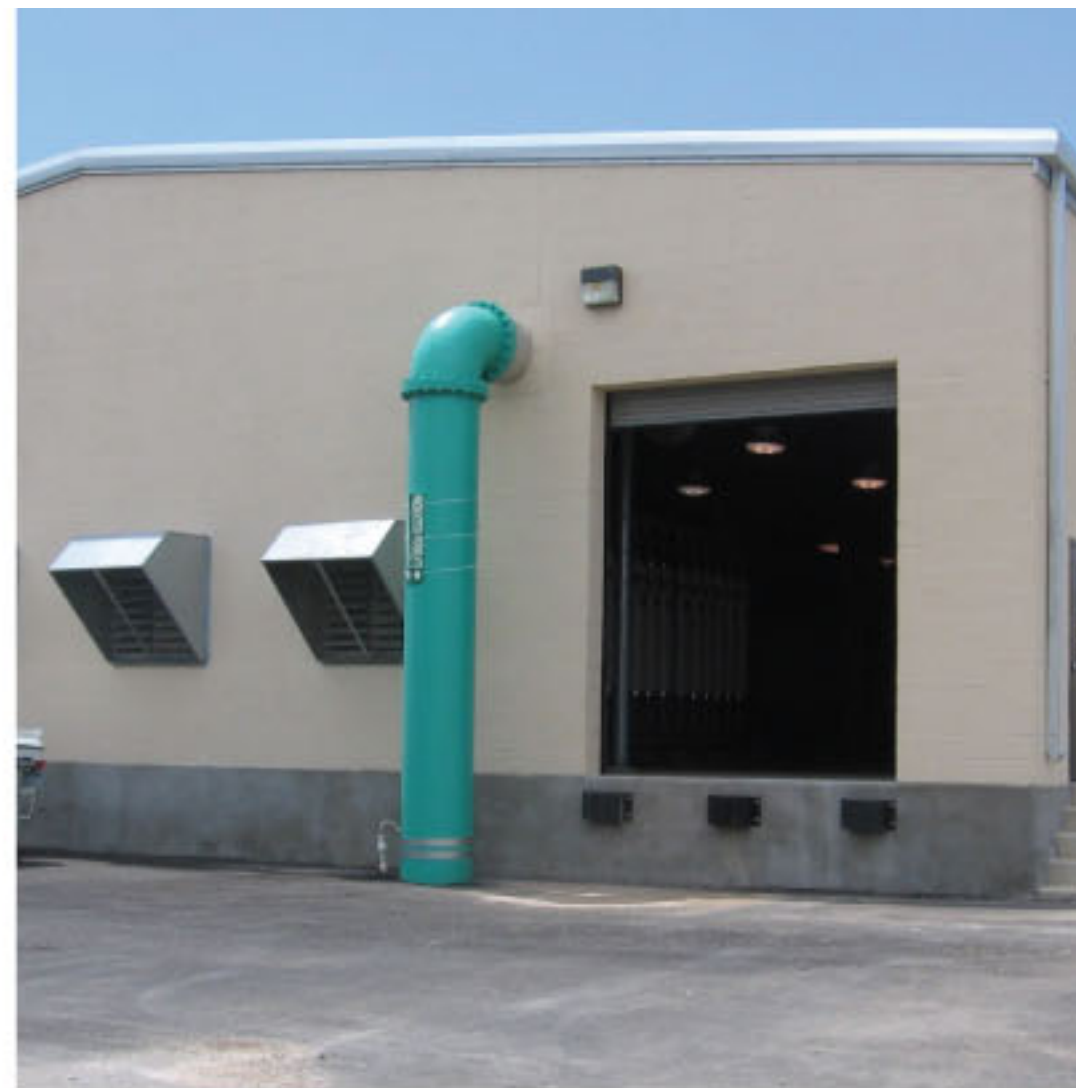
The Lake Dunlap Water Treatment Plant is owned by the CRWA and is located in New Braunfels, Texas. It is one of the many drinking water plants that have turned its attention to membrane filtration.
