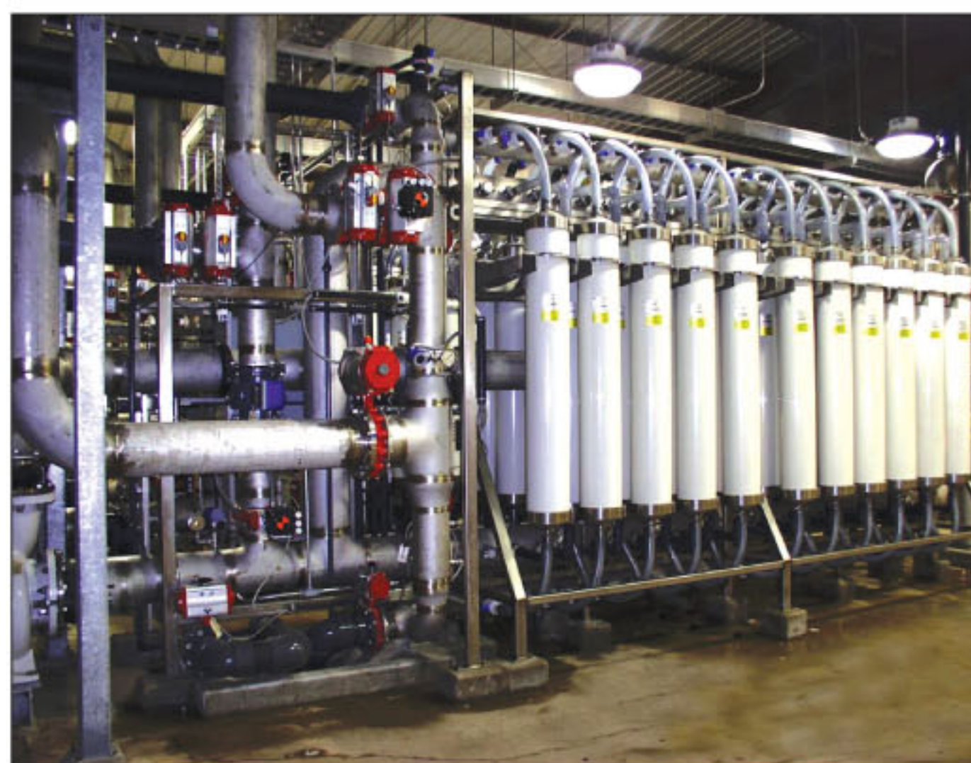
The PMPW ultrafiltration cartridge unit above from KMS is a certified NSF-61 compliant 10-inch diameter hollow fiber cartridge for potable water treatment.
