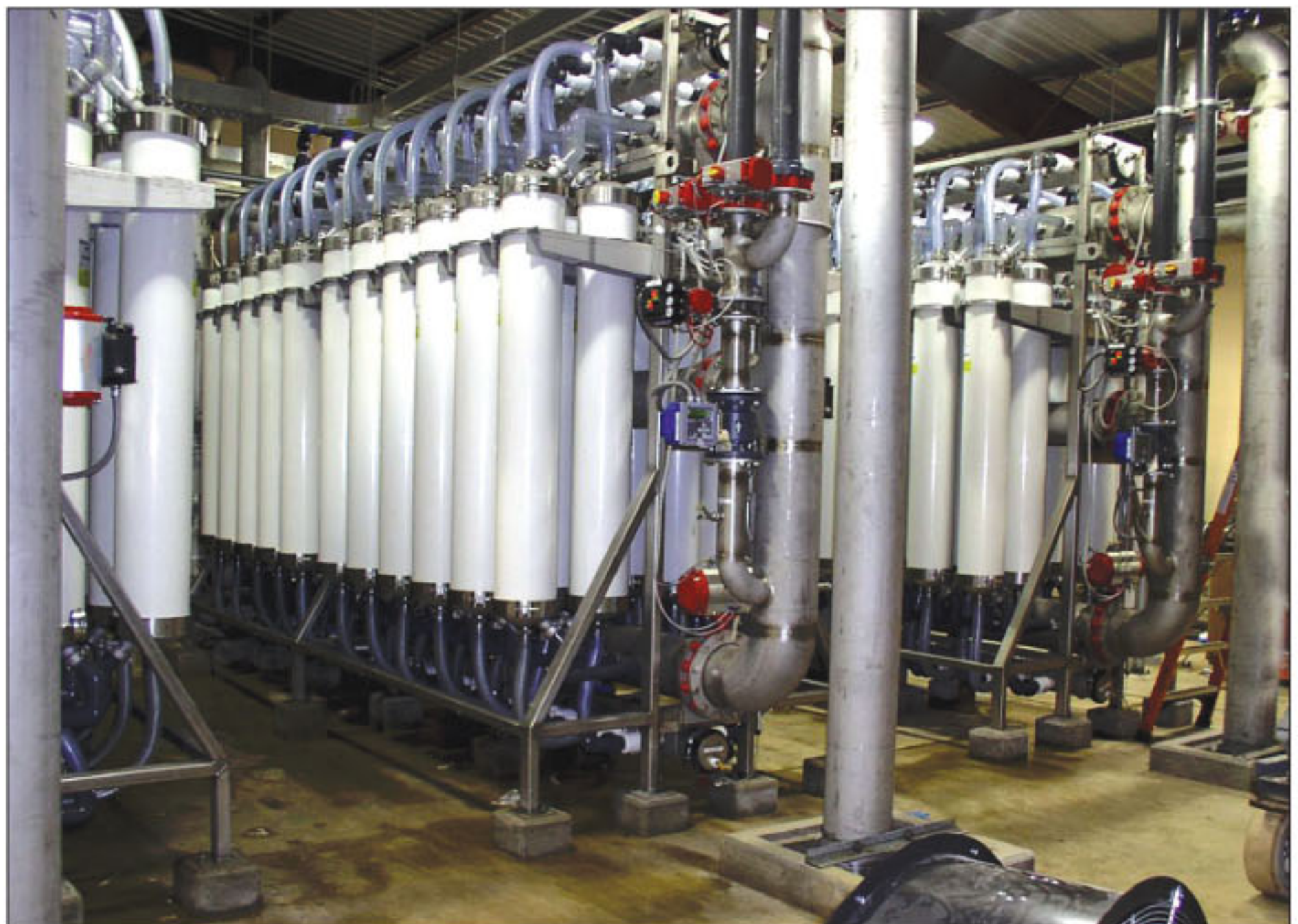
Hollow-fiber filled ultrafiltration cartridges pictured above remove turbidity and provide potable water for the surrounding communities.
